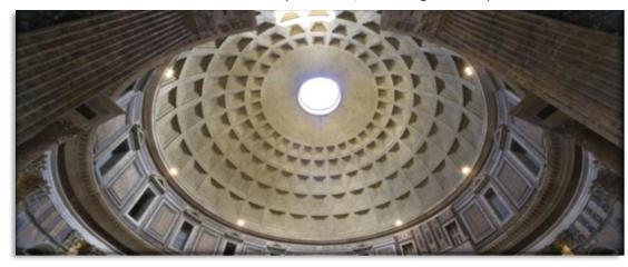
water, the two materials can react to produce strong concrete. But that, as it turns out, is not the whole story. An international team of researchers led by the Massachusetts Institute of Technology (MIT) found that not only are the materials slightly different from what we may have thought, but the techniques used to mix them were also different. The smoking guns were small, white chunks of lime that can be found in what
